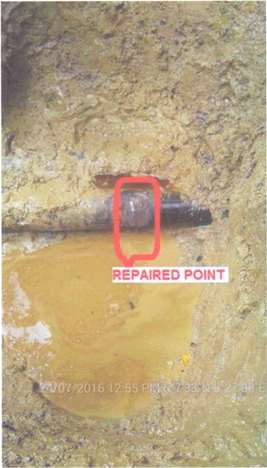
Repaired point Seven (SP7)
